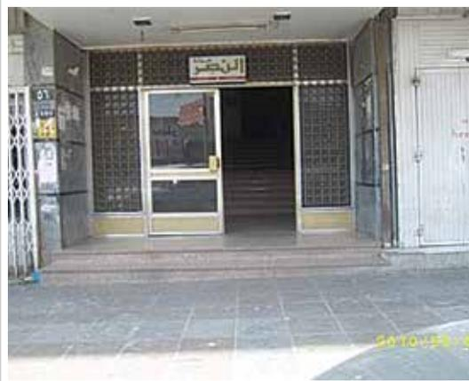
Figure 3. Lack of ramp in a residential building
